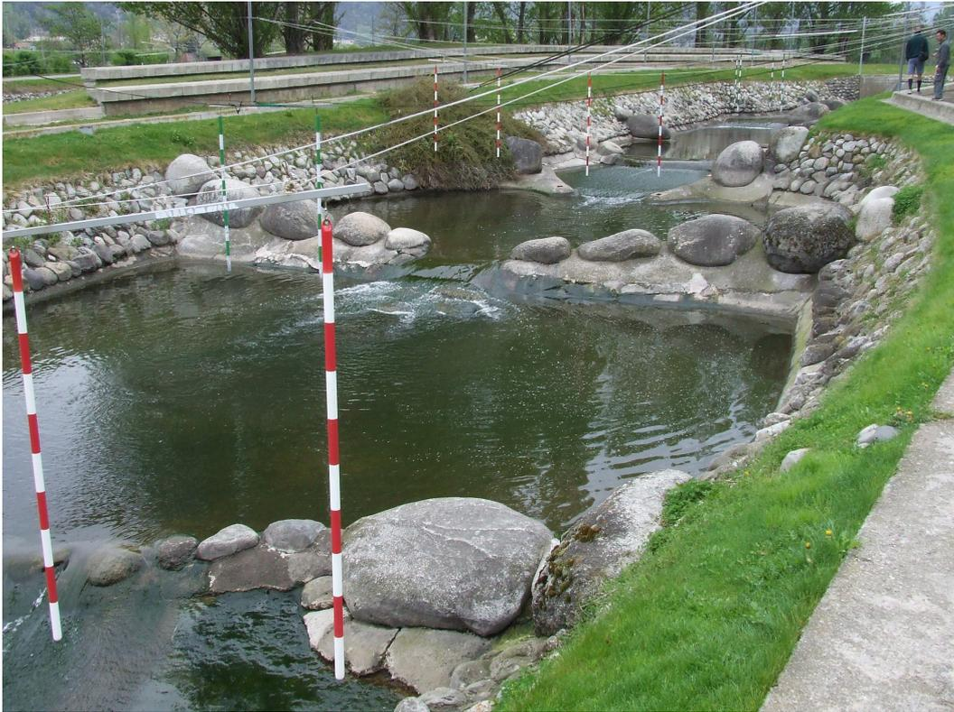
Fig 4-1: Artificial channel for sportive use in Spain in dry conditions.  $15 \text{ m}^3/\text{s}$  of water are pumped at maximum discharge.
