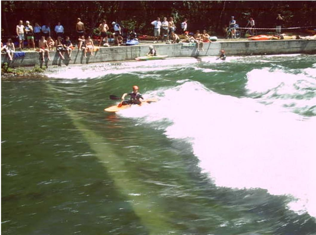
Fig 4-3: Step undular jump in Naviglio channel (Turbigo, 2005)
